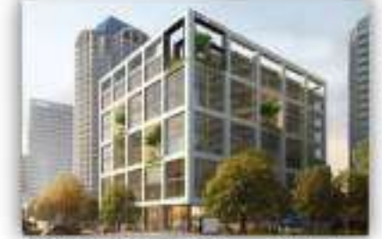
Related Group New Headquarters Office
